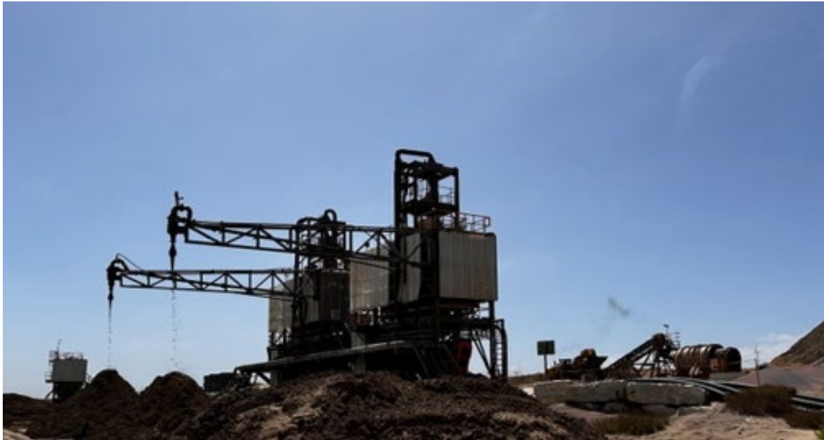
Figure 3 Front-end Processing of Inland Strands Ore (scrubber - background on right, trommel - background left, PBC/TSP gravity separation plant - middle)
